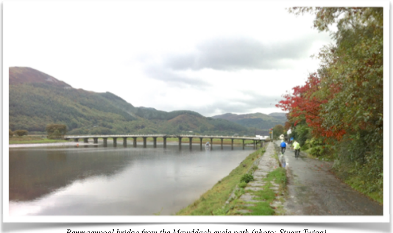
Penmaenpool bridge from the Mawddach cycle path (photo: Stuart Twigg)
